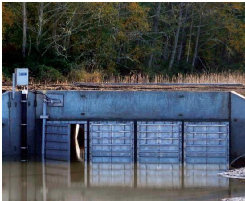
Figure 5-1: Side-Hinged, Passive Hydraulic Activated Gate
