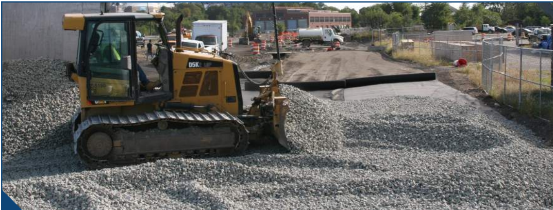
FIG. 2: Spreading and compaction of UL-FGA with a dozer.
