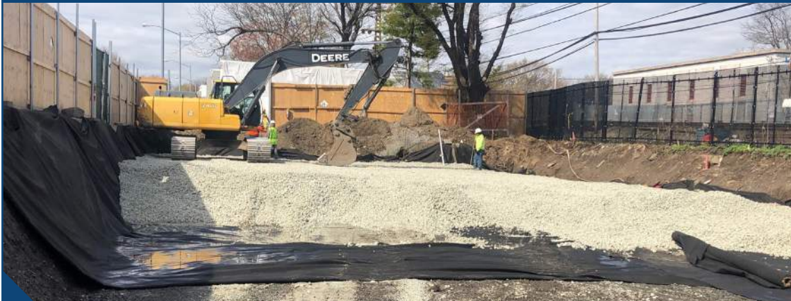
FIG. 3: Compaction of UL-FGA with an excavator.
