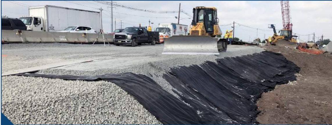
FIG. 4: Placement of capping material on UL-FGA.
