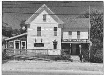
Main Street. Fully renovated year-round building w/ 2 apts. and 2 turn-key businesses. Many original features. Harbor views. Possibilities! $749,000
