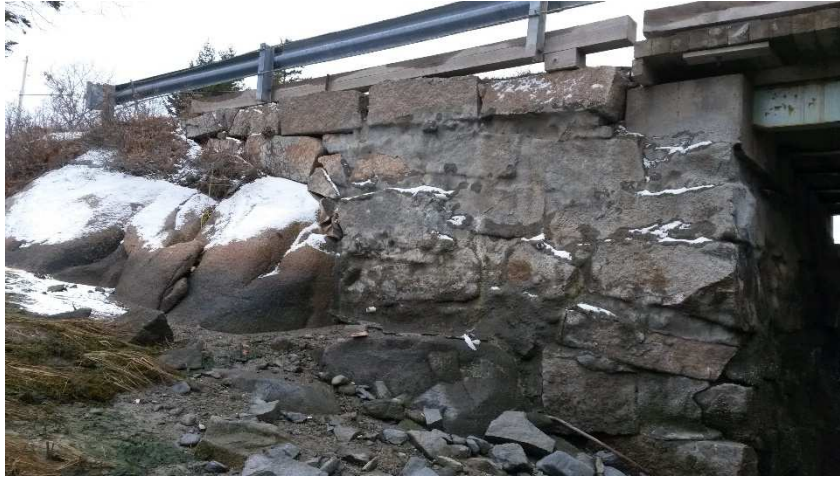
Granite Block Cribbing (Portions with Shotcrete) – Southwest Abutment
