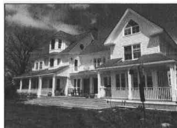
Leo's Lane. Fabulous 5 bdrm, 3 bath home, w/ ocean views and deeded harbor access. Excellent craftsmanship and impeccable details. $769,000
