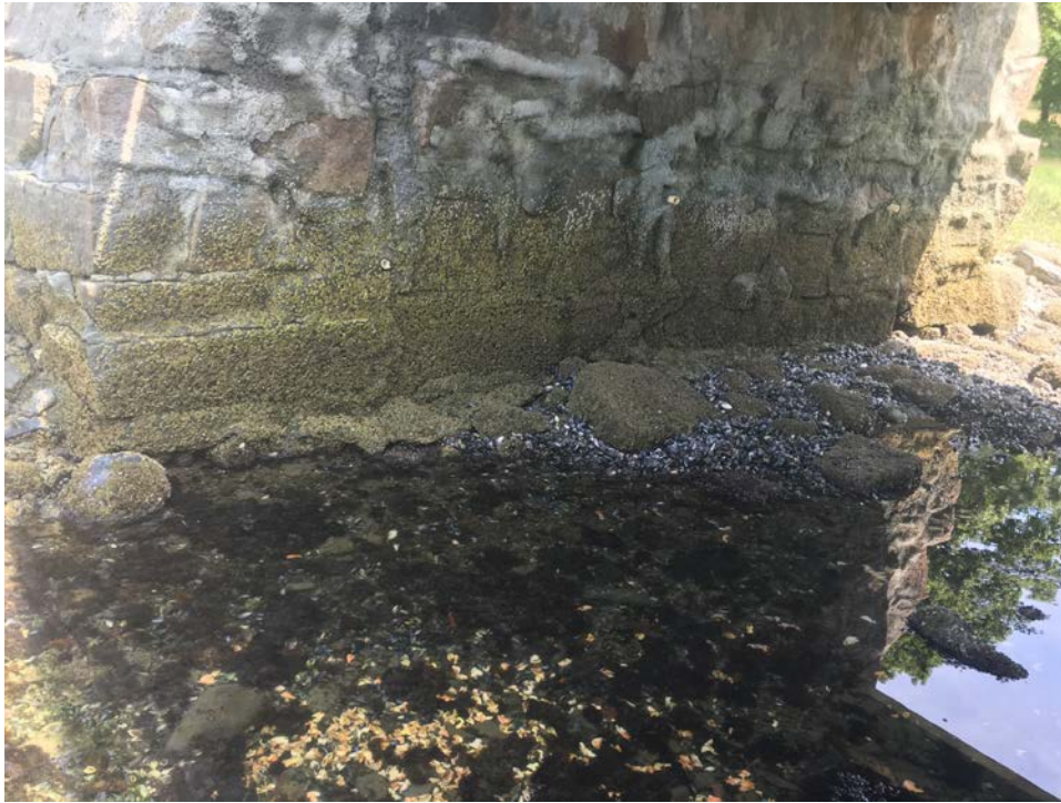
PICTURE 9: Toe of Abutment and Bed Substrate
