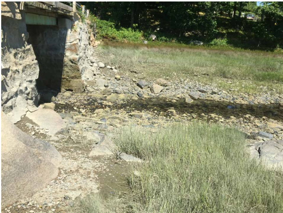
PICTURE 10: East Side of Abutments and Adjacent Bed Substrate
