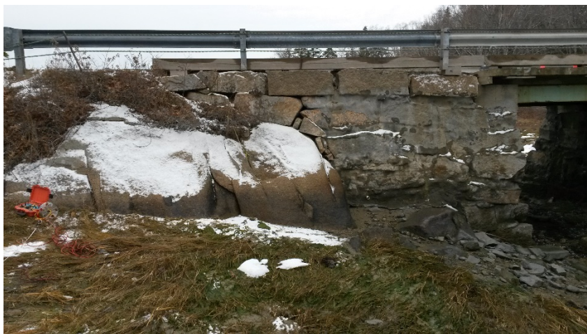
Southwest Abutment – Dipping Ledge to Mud/Ledge to Cobble Channel
