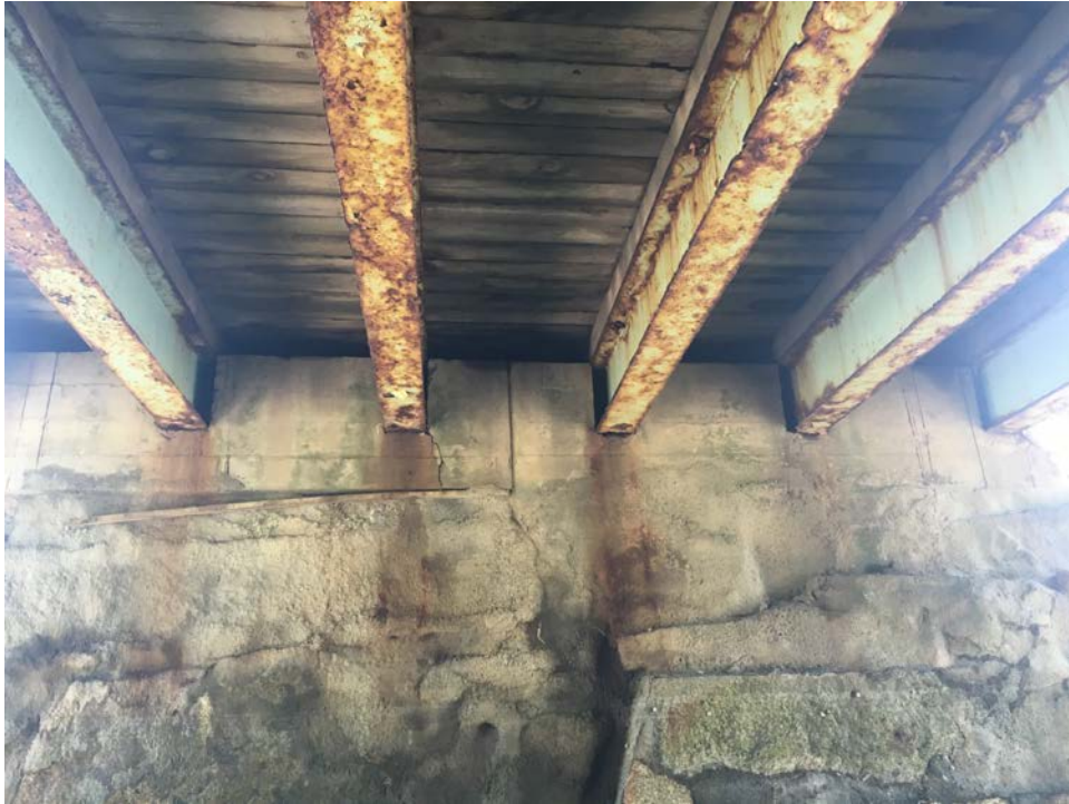
PICTURE 7: Northeast Abutment, Steel Girders and Timber Deck
