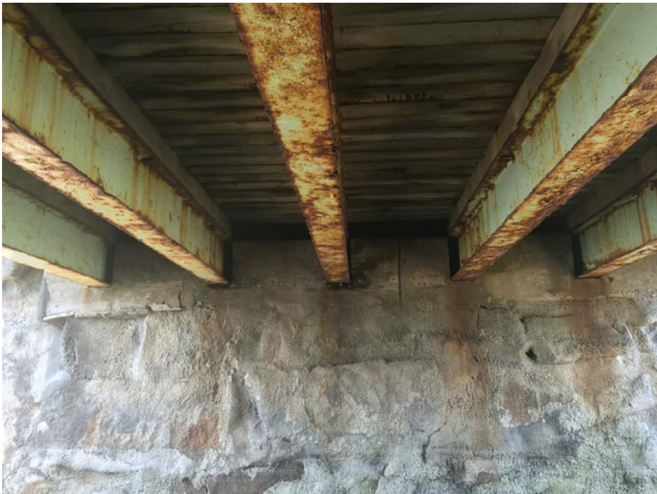
PICTURE 8: Southwest Abutment, Steel Girders and Timber Deck
