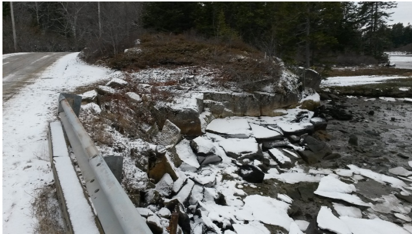
Southeast Abutment – Steep Bedrock to Mud to Cobble Channel
